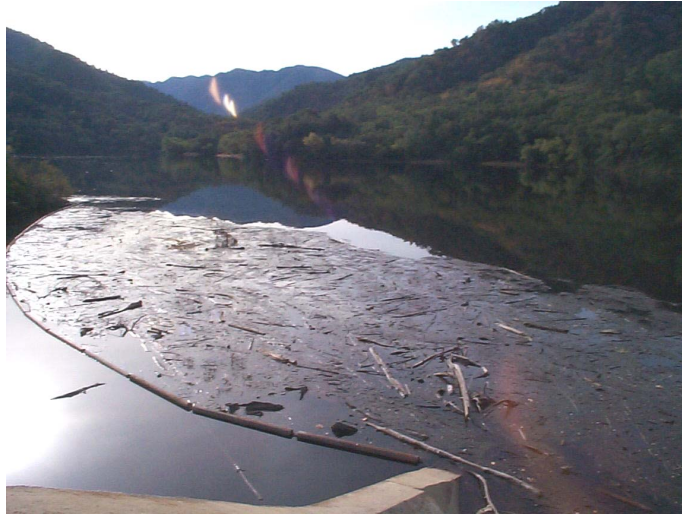
Figure 5.5.1.5-C. Picture of Los Padres Dam log boom taken on 11/15/2002.
